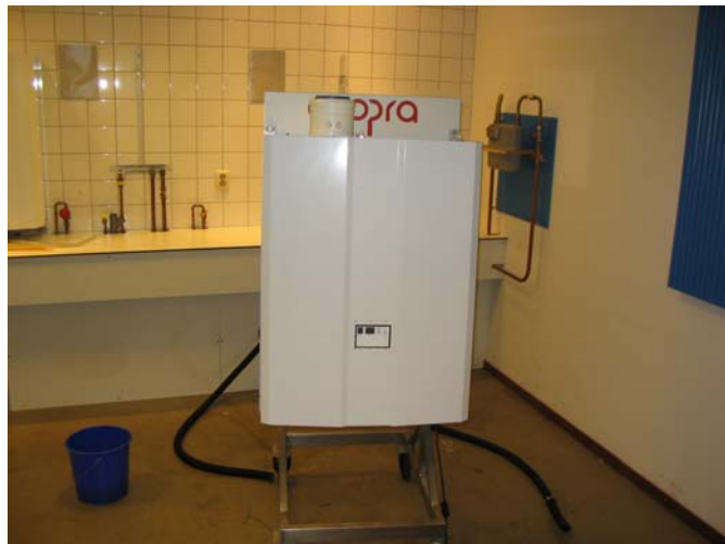
Wall hung, fan flue, room sealed gas boiler
